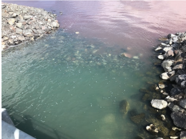
Figure 4. The breach showing the raised adaptive management berm blocking the return flow of saturated brine from the North Arm (pink color)
