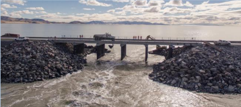
Photo by Ames Construction, general contractor of the project
